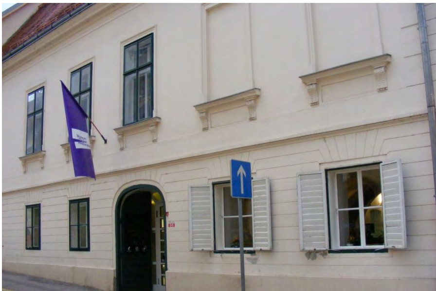
Figure 1:1 Museum building, 2 Sv. Cirila i Metoda Street, Zagreb
