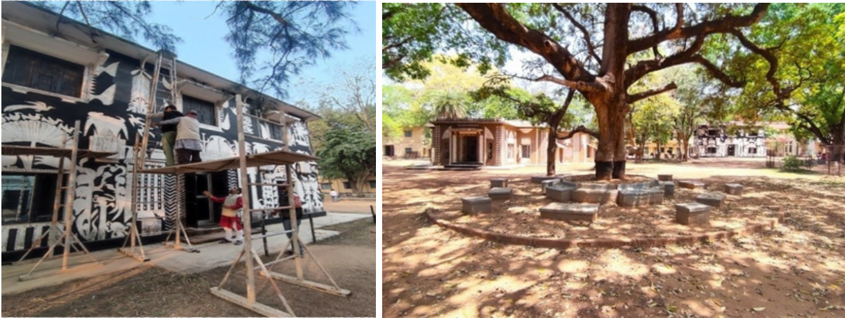
Fig 9: (left) Department of History of Art on the left and the Department of Design on the right, inside Kala Bhavana Campus. Source: Author, 2024; (right) K.G. Subramanyan's Black and white Mural on the walls of the Design Department, Kala Bhavana. Source: Author, 2024.
