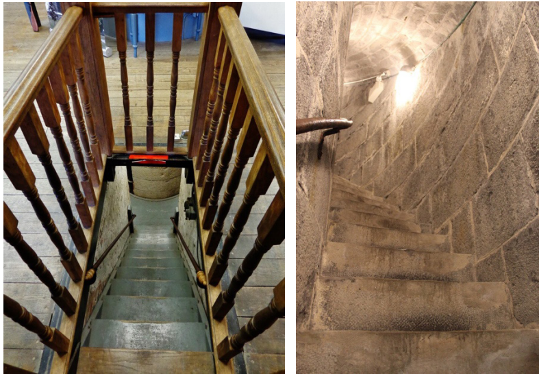
Figure 4. Interior stairs going into the basement (left) and the gun platform (right). Photo Collection of the Murney Tower Museum, 2021.
