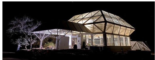
Figure 1 – The Space Analog for the Moon and Mars biodome. An Earth based biodome to replicate the conditions of living on an extraterrestrial body to validate the systems and technologies to be used on the moon and Mars [3].
