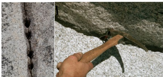
Figure 1 – Pitons are designed to be hammered into cracks to provide protection to climbers, because of this they are intended to be very hard to remove. Removal of pitons causes rock scarring as the surrounding rock must be removed as well.
