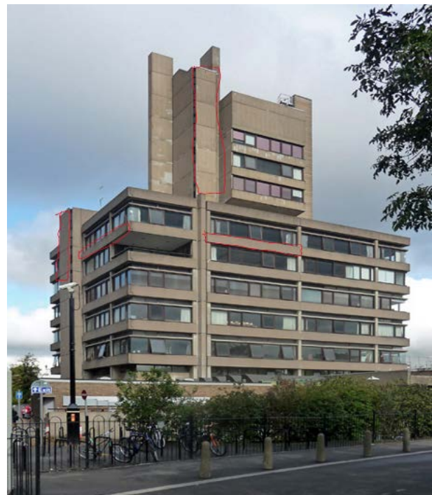
Figure 1 – Photo of the Charles Wilson building. In red are examples of the concrete blocks counted to carry out calculations [2].
